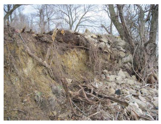
Plate 3. A section of the Army Creek Dike bank eroded from the effects of Hurricane Sandy.
