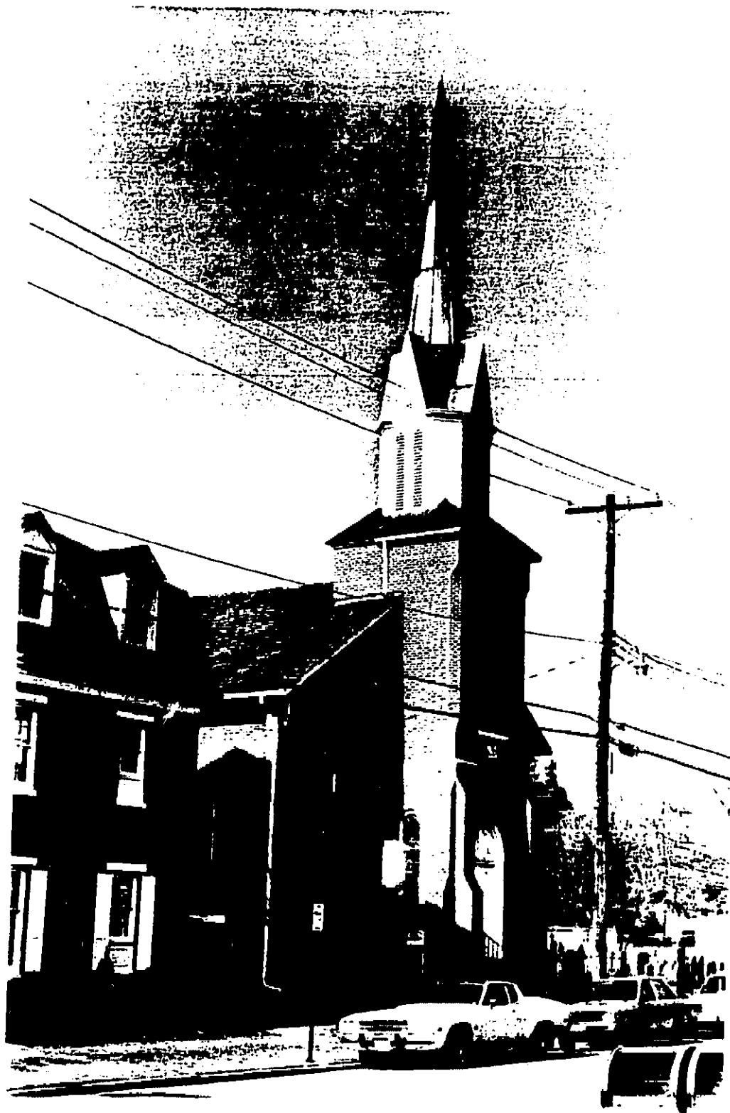
N. 549. 494 New Castle Methodist Church 510 Delaware St.
