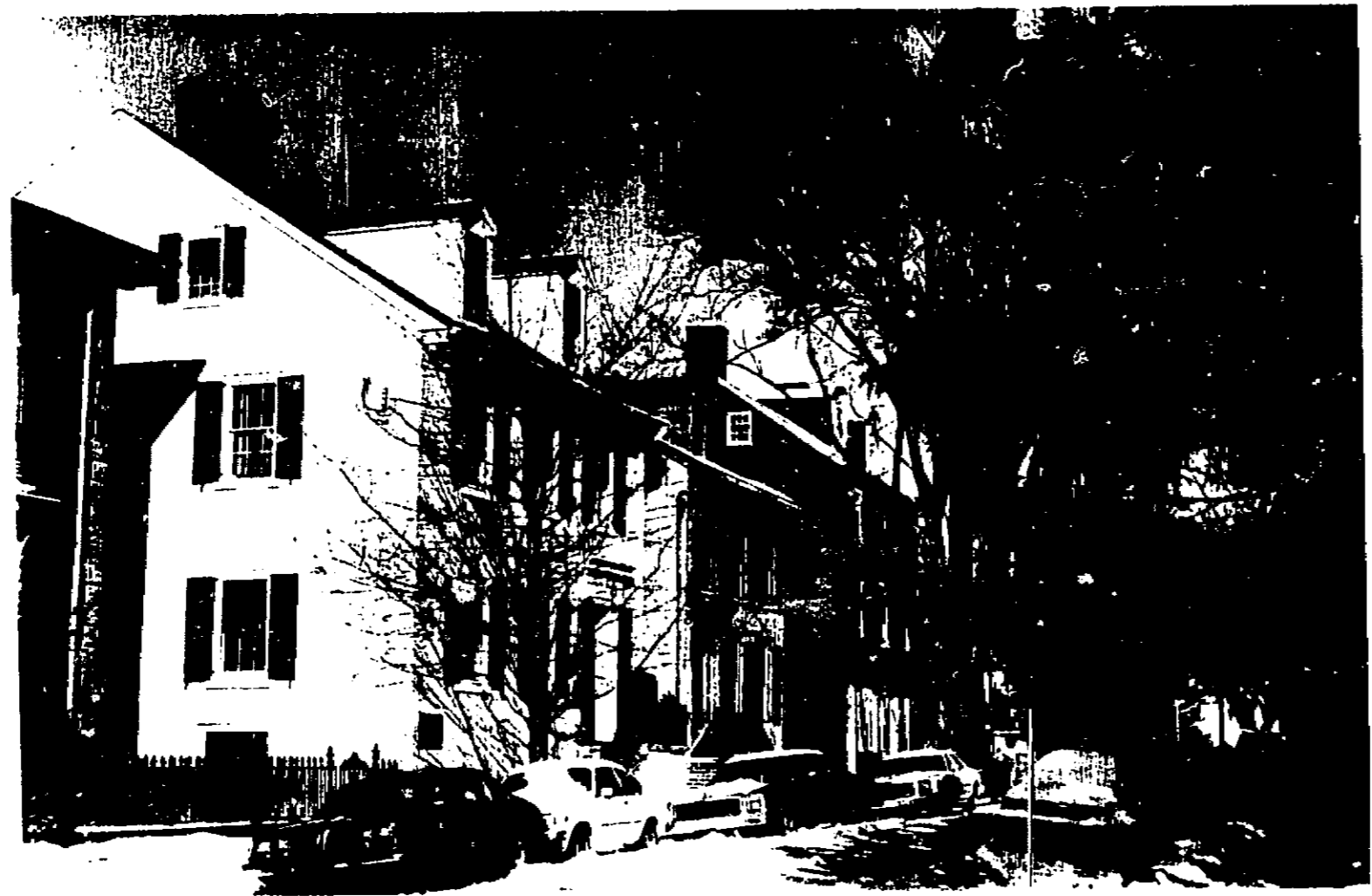
N-349. 19 GUNNING BEDFORD HOUSE 6 THE STRAND
