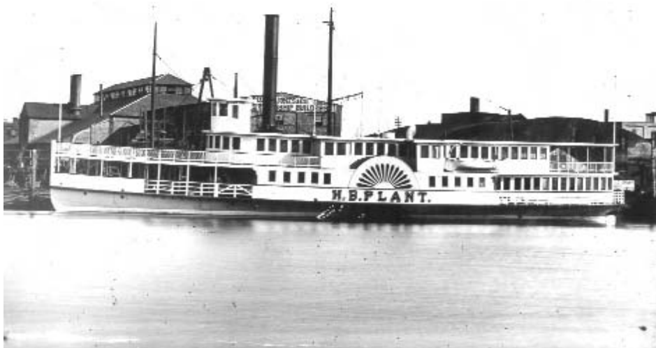
Figure 5. The Steamship H.B. Plant at Pusey and Jones Shipyard in Wilmington. This shipyard was flooded with at least a foot of water in the buildings (Courtesy Hagley Museum and Library).
