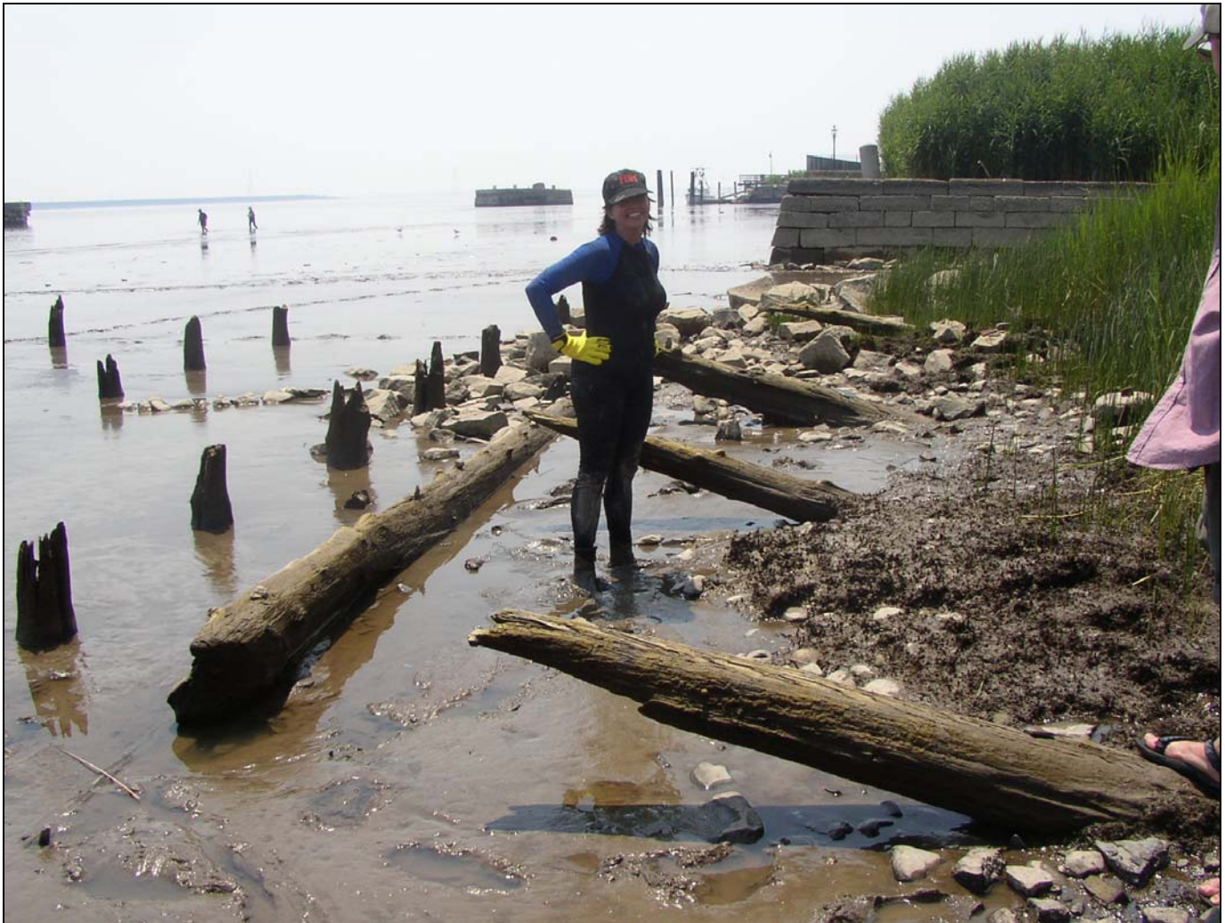
Figure 37. The shore timber assembly looking downriver to the south. The inner ice pier "G" at the end of Alexander Alley is seen to the upper right of the field. Note the horizontal and diagonal wharf timbers.
