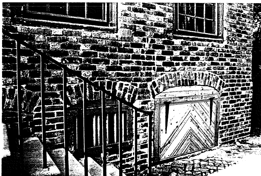
View of cellar window openings
