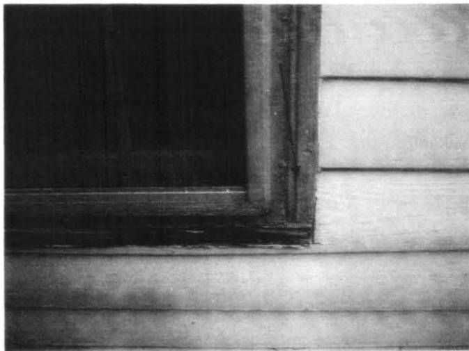
Showing a window sill in need of replacement.
