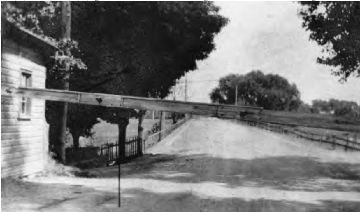
Tollgate on the old Kennett Pike. The Wilmington & Kennett Turnpike opened in 1813. It was Delaware's longest operating turnpike when the gates were removed in 1919 and the road turned over to the county as a free road.
