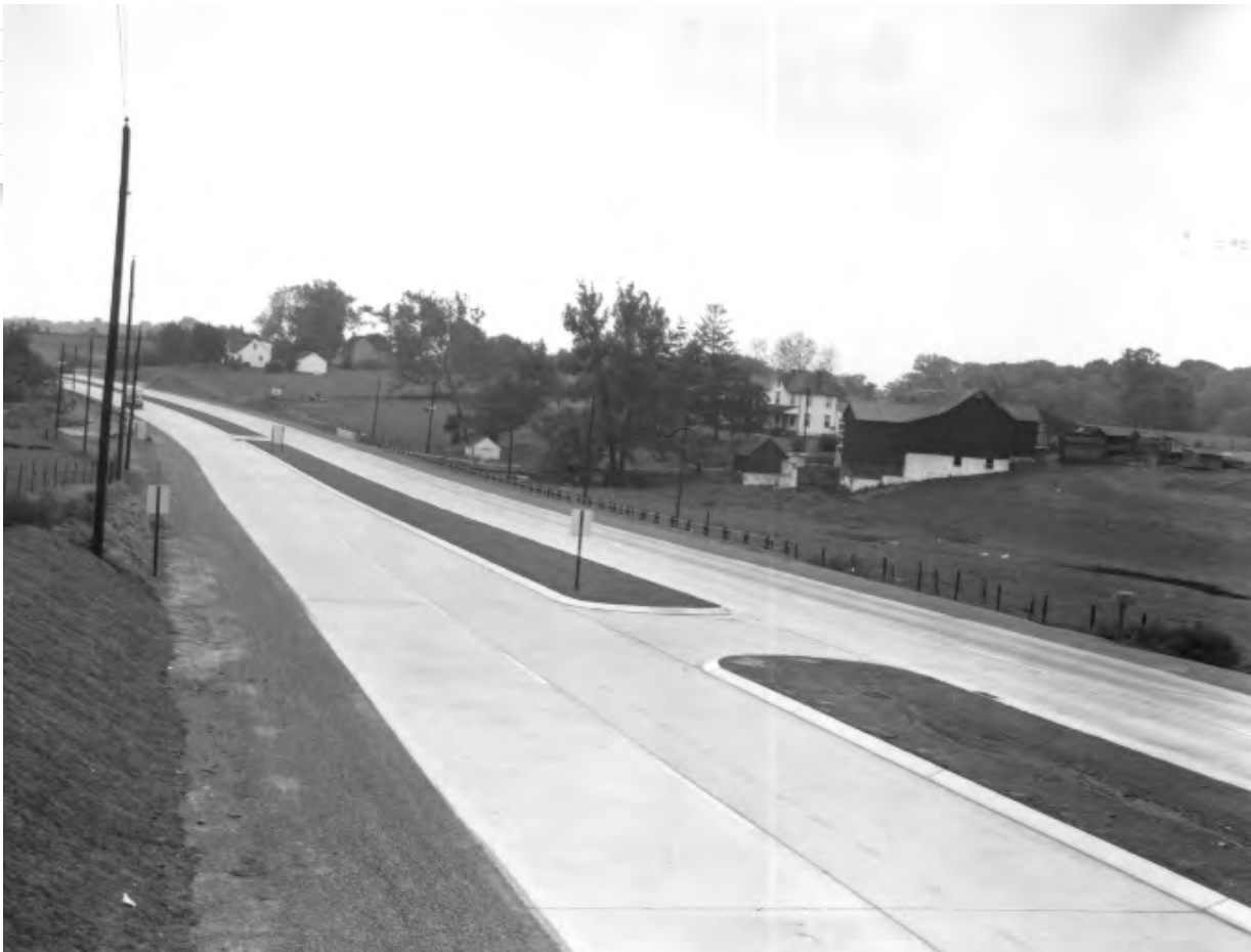
The Concord Pike (US 202) was one of many Delaware highways dualized for greater capacity in the 1950s.
