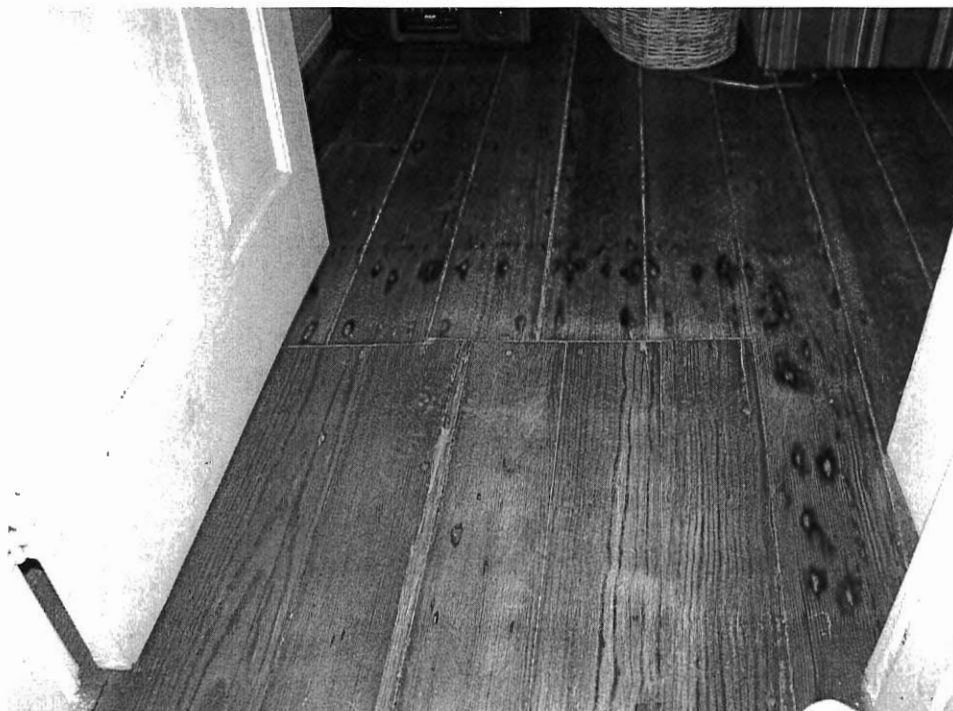
Figure 7: (left) Patch in front of cellar stairs indicating original winder stair.
