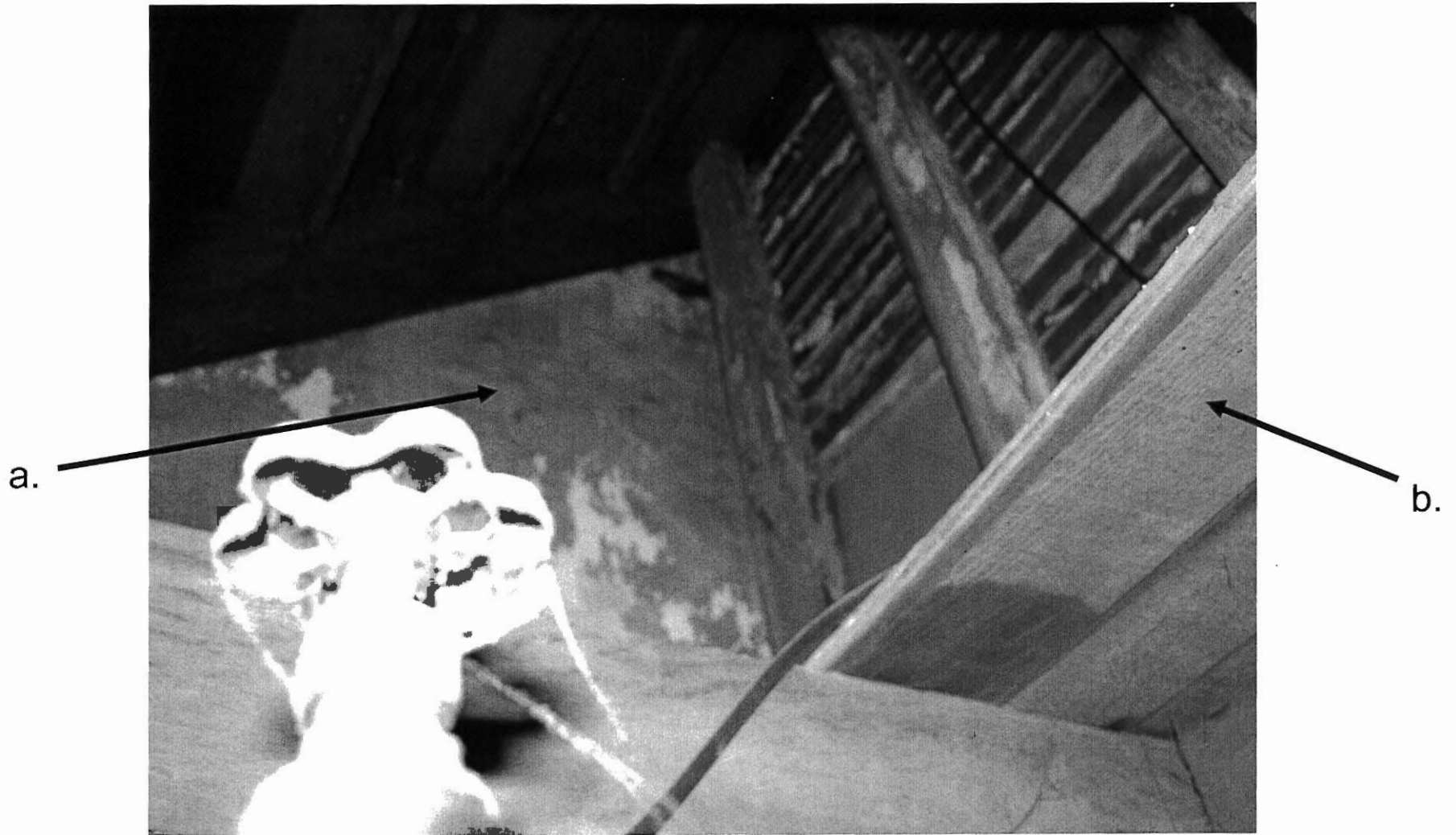
Figure 6: Evidence of plaster (a) on rear wall under modern stair in front room. Notice also the floorboards (b) that extend from the front room, through modern wall to original back wall.
