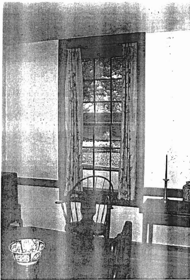
Fig. 15 View of the first floor back room (Dining Room) Note how the chair molding wraps around the bottom of the window sill.
