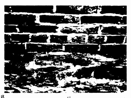
A. Front elevation, Flemish bond B. Side elevation, common bond, rubble foundation
