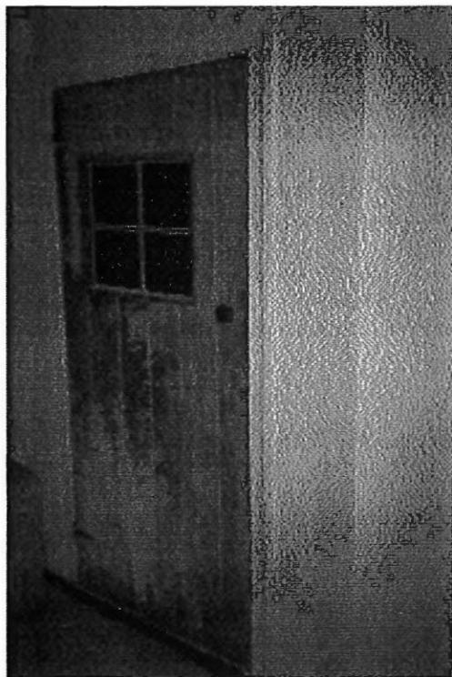
Fig. 24 Weathered door now used for closet in cellar
