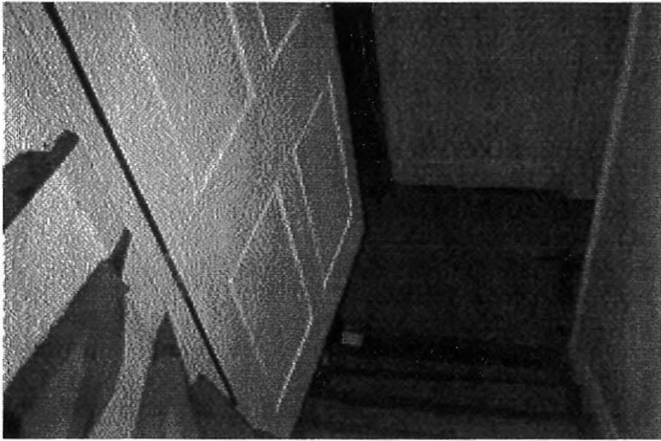
Fig. 13 Stair leading to attic
