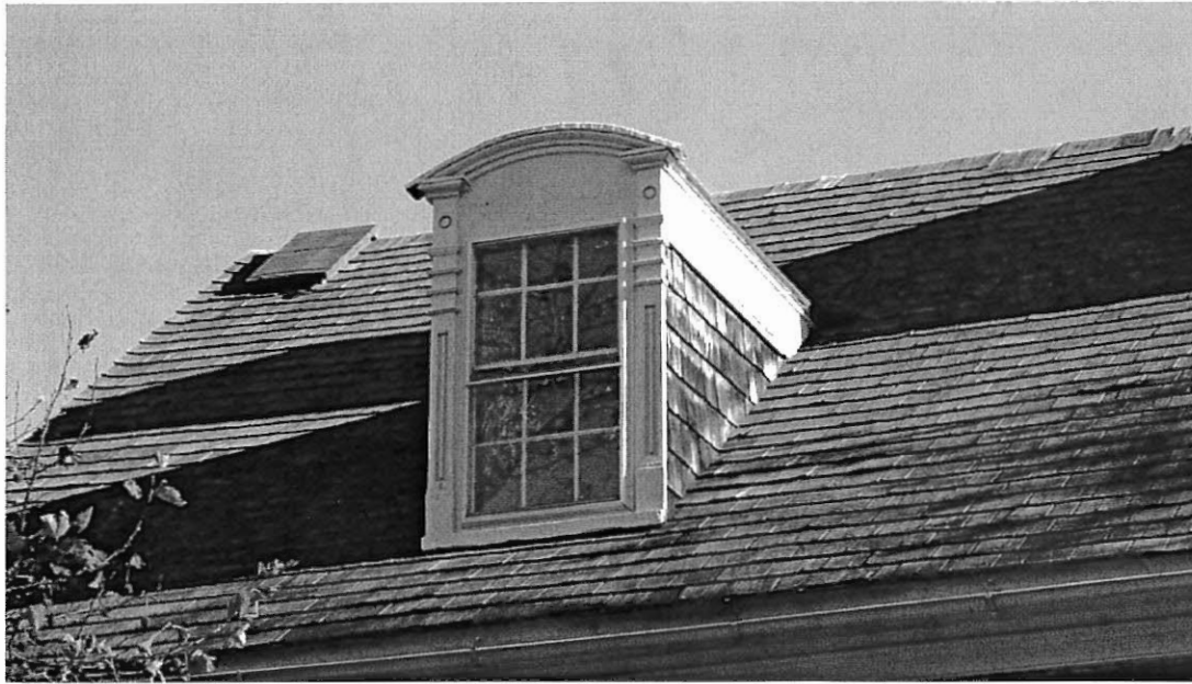
Figure 3. Front dormer window and attic trapdoor.
