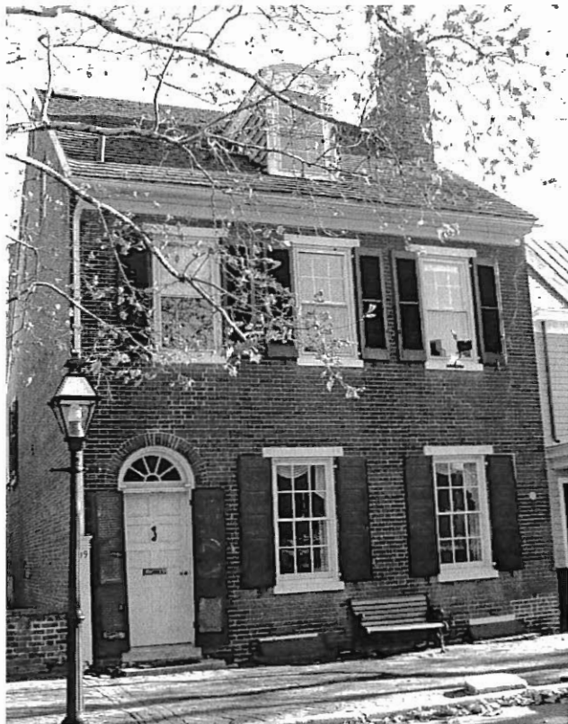
Figure 2. Front façade of 19 E. Second Street.
