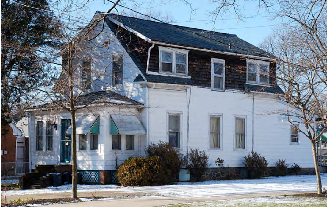
Figure C.2 Order 4400, Portland #1, G. P. Weatherlow, perspective of east and north elevations, 207 Beeson Ave, Edgemoor. (Source: Photo by author, December 2009.)
