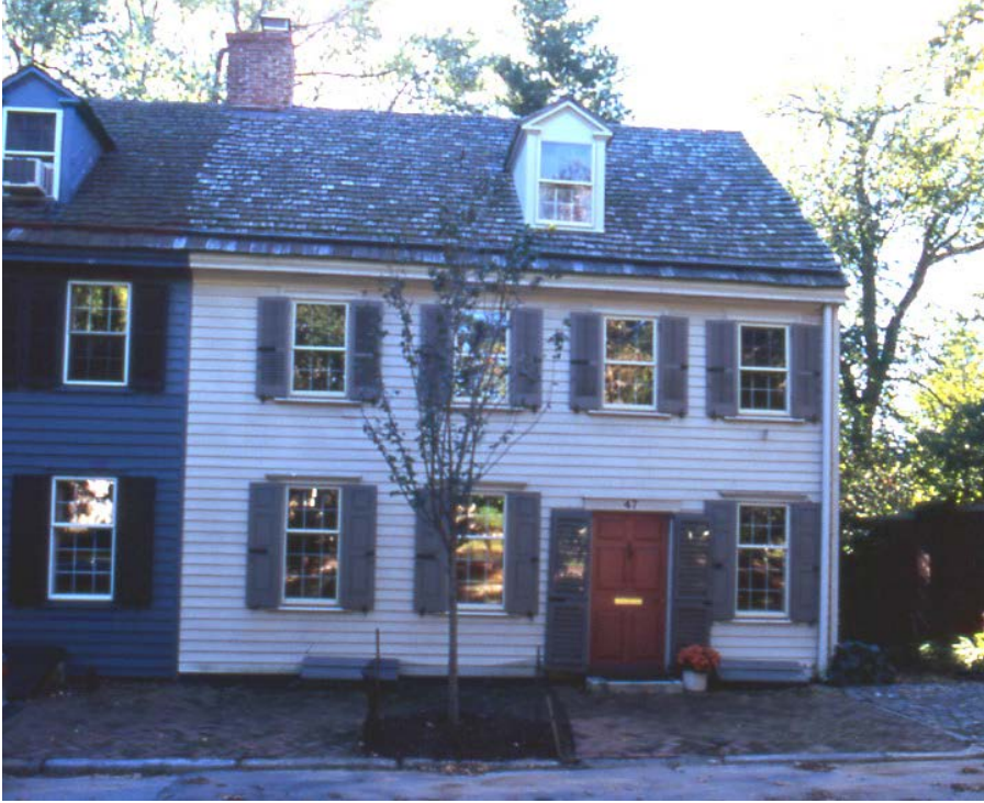
Fig. 1. Aull House, 47 East Second Street, New Castle, DE
