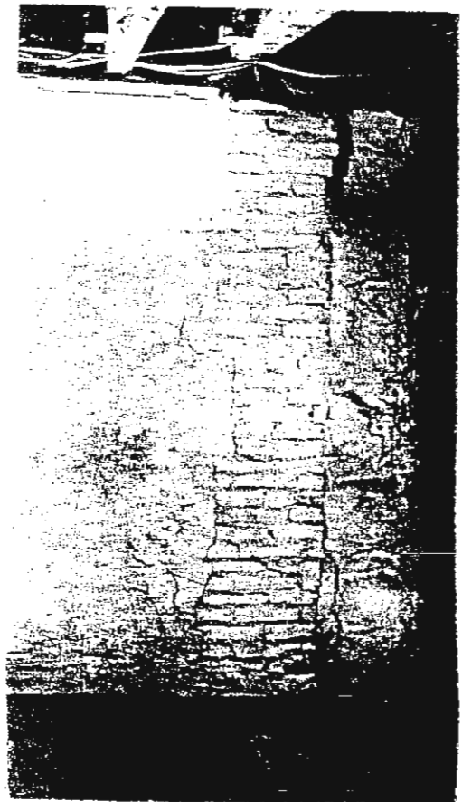
Fig.1. Interior of bricked doorway, photo from Natl. Reg. p5
