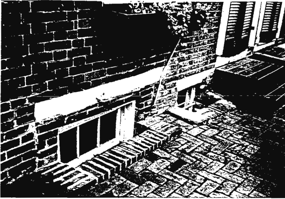
Fig. 2. Exterior of bricked entry to basement.
