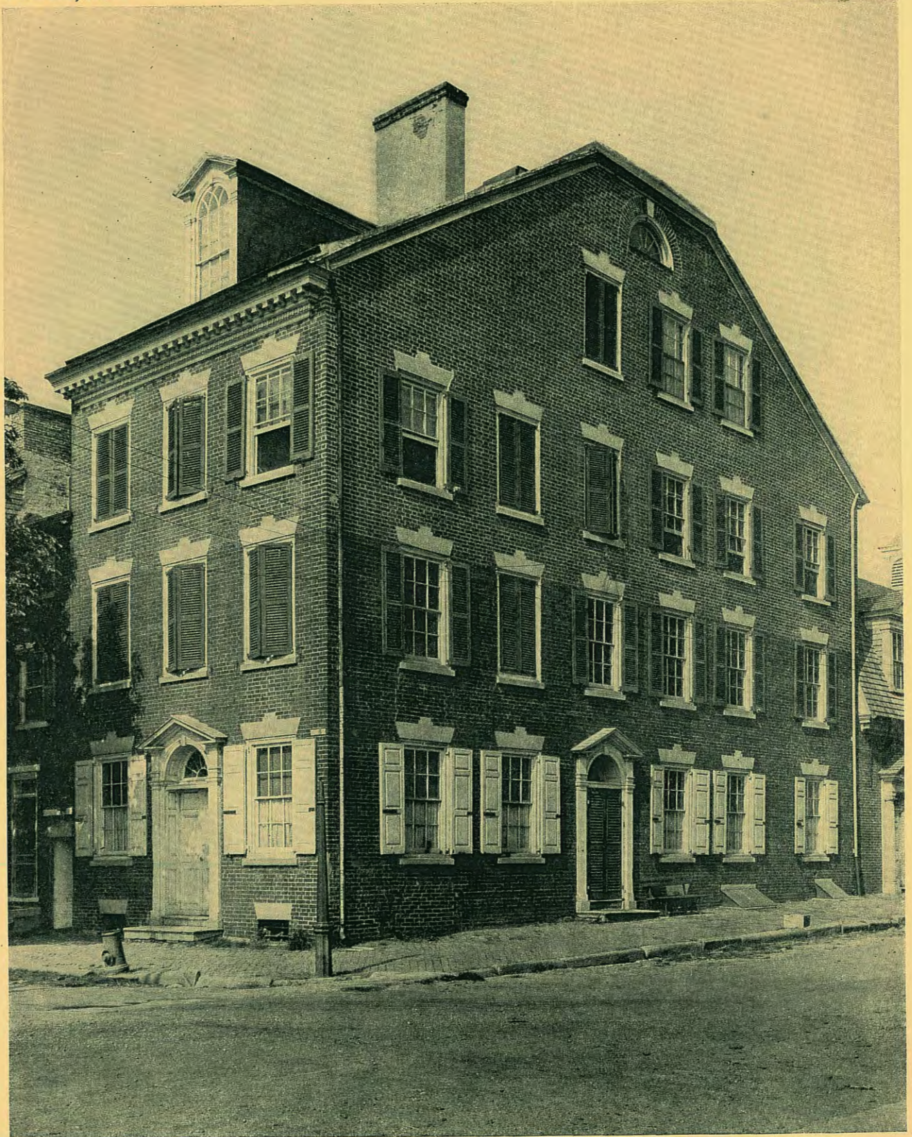
THE CHARLES THOMAS HOUSE, NEW CASTLE, DELAWARE (Built about 1801—Now called "The Parish House")
