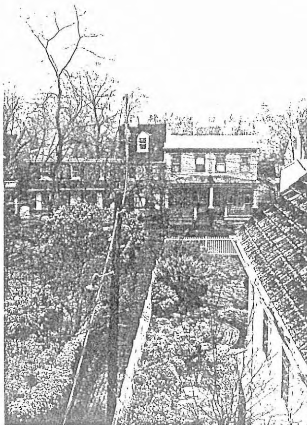
Fig. 26. View from rear chamber on second floor.
